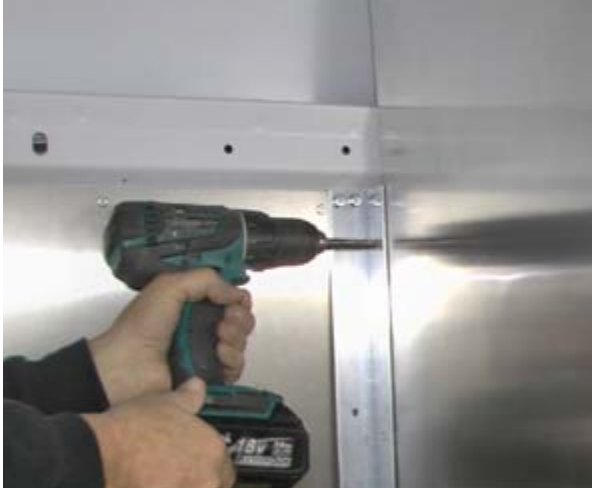
Holes drilled in angle and LH bulkhead wall
