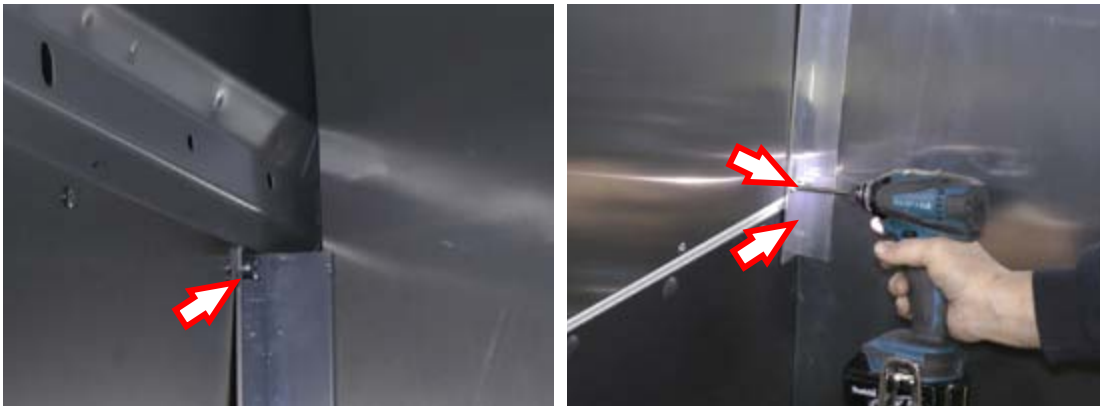
Screws in upper and lower vertical angle
