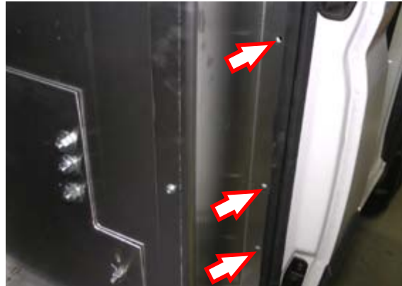
Closeout panel holes
